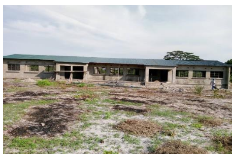
Uncompleted 1x3 CRB at Nakatondo Community School
