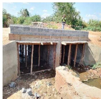
Dambo road Culvert under construction
