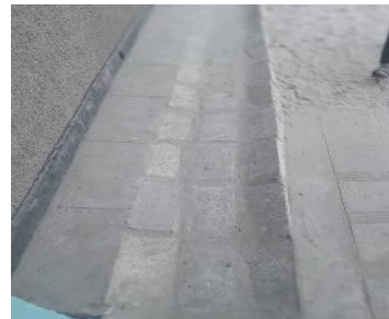
Front view of 1x2 CRB at Mabumbu School Shoddy works on the spoon drain
