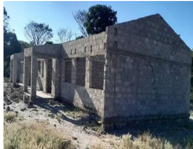
Incomplete 1x3 CRB
