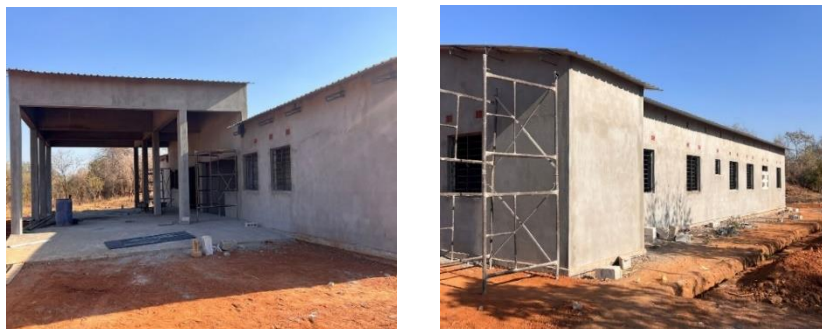
Incomplete Rural Health Post
