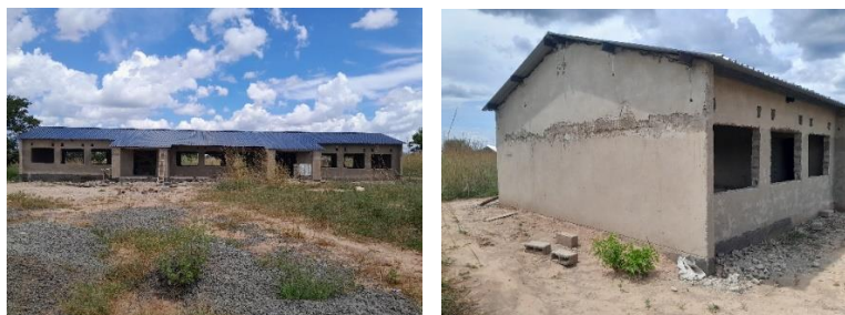
Uncompleted 1x3 CRB at Kaloli Community School
