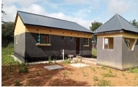
Staff House without power connection
