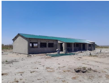
Front view Nakaya Primary School
