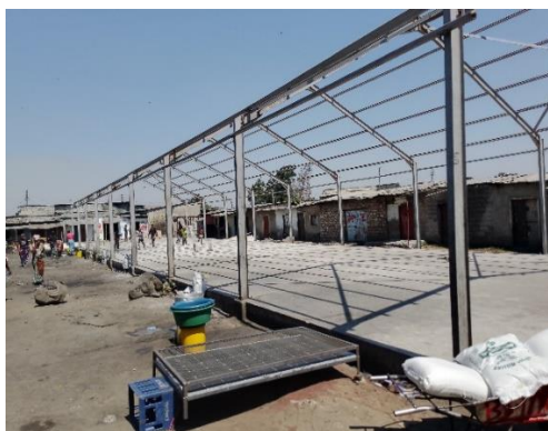
Incomplete Traders Shelter
