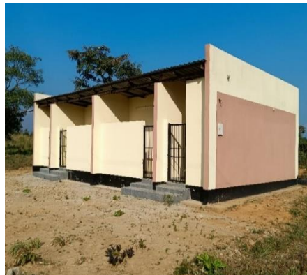
Newly constructed ablution block
