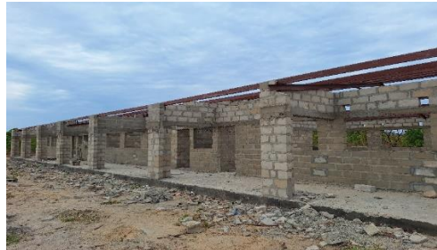
Uncompleted 1x3 Classroom block at Chileng'a Secondary School
