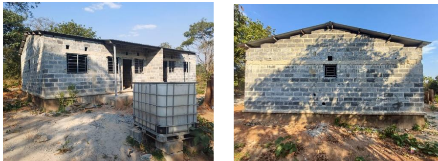
Incomplete semi-detached house at Milulu
