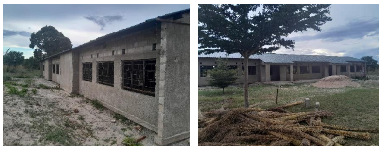
Uncompleted 1x3 CRB at Kashinzi Community School
