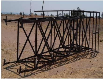
Water tank still not erected
