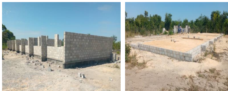
1 st 1 x 3 CRB at ring beam level
