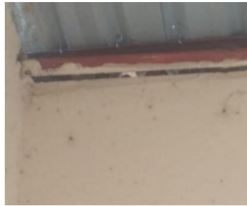
Truss Separated from the Wall
