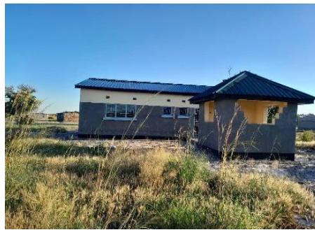
Incomplete staff House and Kitchen
