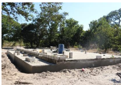
Figure 10 -Slab Level at Nakayembe Maternity Annex
