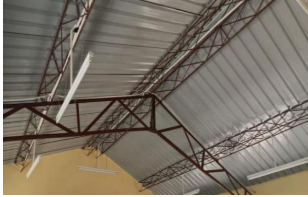
1x2 CRB roof without ceiling board
