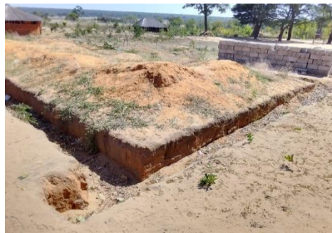
Figure 3-Footing Stage Makumba CRB
