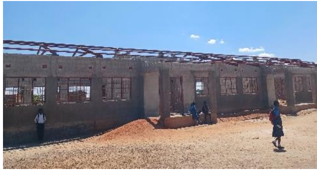
Incomplete 1x3 Classroom Block at Lugwasho
