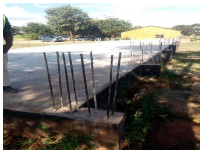
Incomplete 2x3 Storey block
