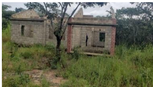
Incomplete staff house
