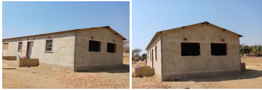
Incomplete Staff House at Siasikabole Primary School
