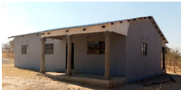
Incomplete Staff House at Munteмба Primary School
