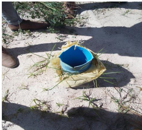
Vandalised casings at Mukalizi Primary School
