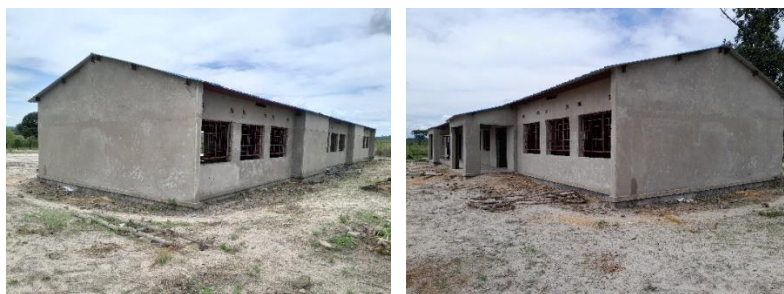
Uncompleted 1x3 CRB at Njatanga Community School
