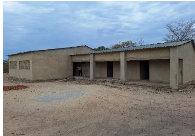
Uncompleted Kanunu Health Post
