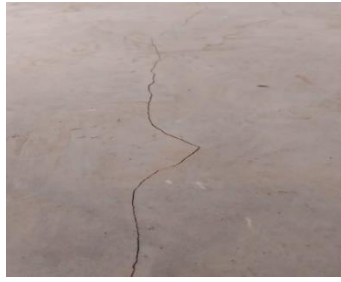
Cracked Floor
