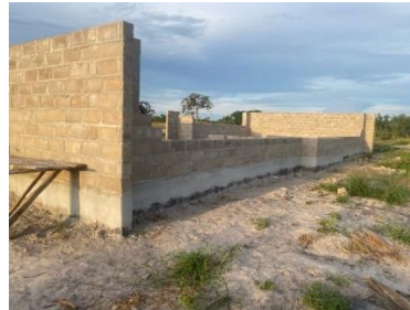
Uncompleted 1x2 CRB at Libinga School
