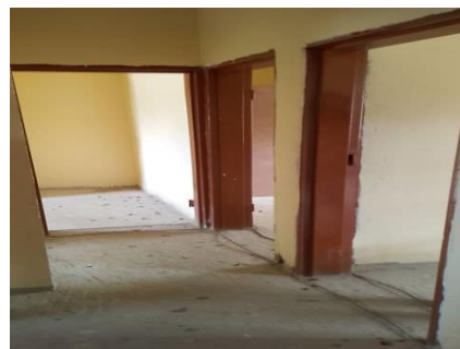
Incomplete staff house
