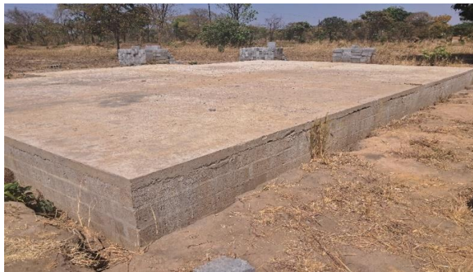
Stalled Police Post at Slab Level
