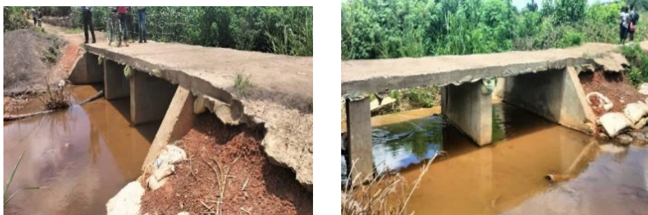
Incomplete Bridge at Mishishi Stream
