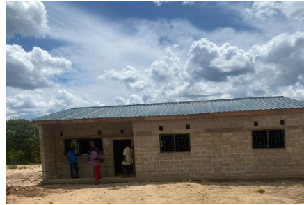
Uncompleted Staff House at Kaoma-Ndonga Health Post
