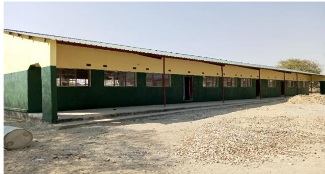
Incomplete 1X3 Classroom Block at Mukamba
