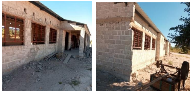
Construction of 1x3 CRB at Samisisi Primary School
