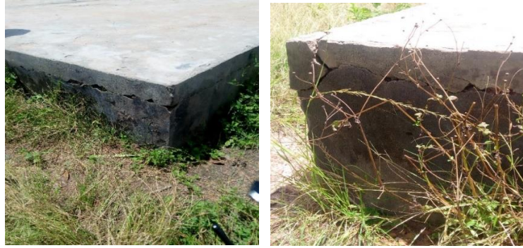
Cracked Slab
