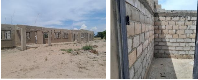
Uncompleted 1*3 CRB at Kaaba Hill Primary School
