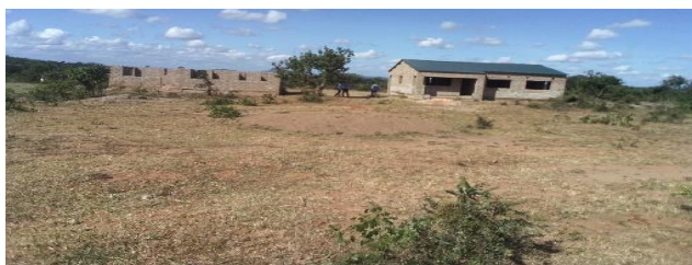
Incomplete Staff Houses at Chibondo
