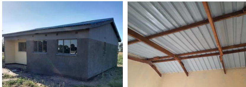
Incomplete staff house
