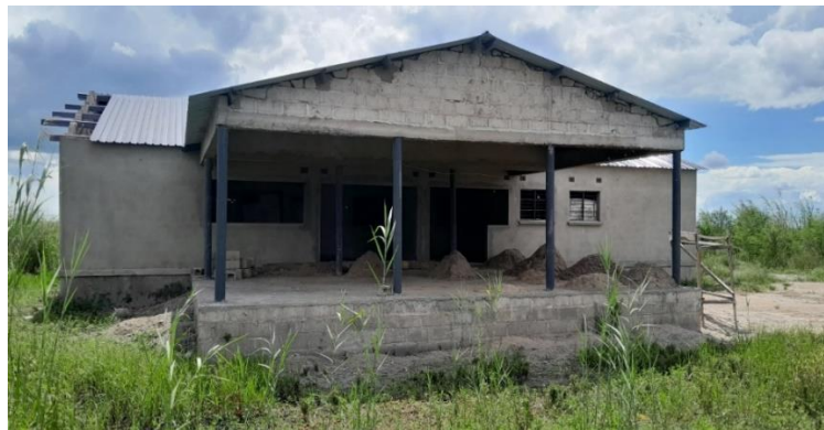
Incomplete Mung'omba Health Post
