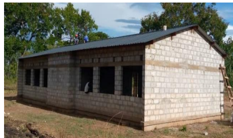
Uncompleted 1x2 CRB at Kajejeje School
