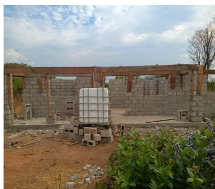
Super structure under construction
