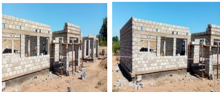
Incomplete 1 x 3 classroom block
