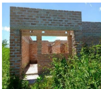
Structure at roof level
