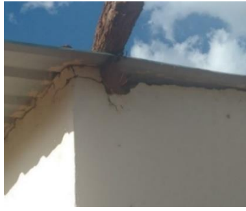
Damaged Roof and Cracked Wall Crack on the Floor of one (1) Bedroom
