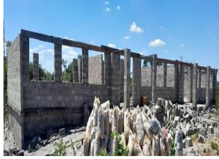
Incomplete 1x3 CRB
