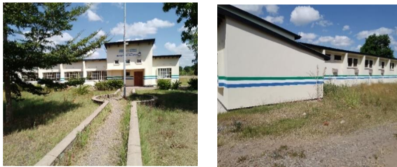
Rehabilitated Police station
