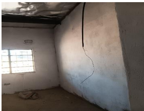
Incomplete Wiring
