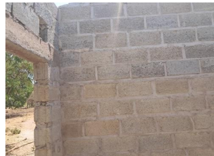
Abandoned Two (2) Bedroom House at Gamble Level Structure Without Ring Beam Inside
