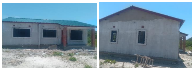
Front view of Kaande Staff House
