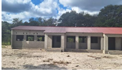
Uncompleted 1X3 CRB at Makwaza Community School
