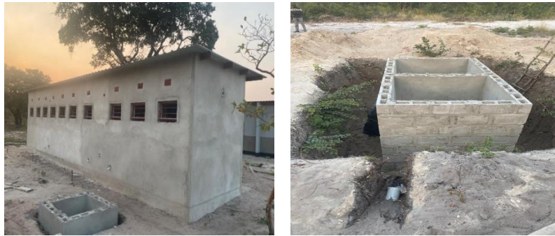
Uncompleted Girls ablution block at Nangula Secondary School
