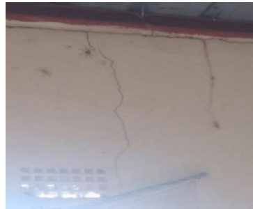
Cracks on the Wall
