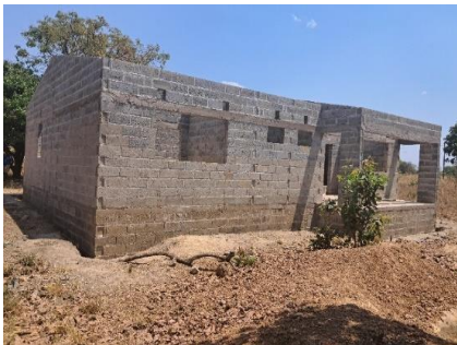
Abandoned Two (2) Bedroom House at Gamble Level Structure Without Ring Beam Inside
