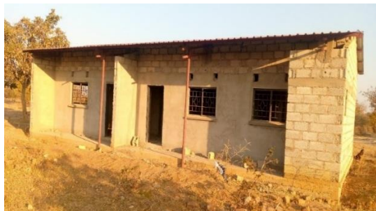
Incomplete Health Post
