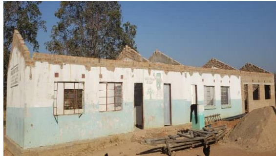
Incomplete 1x3 classroom block at Shimbunji Community School
