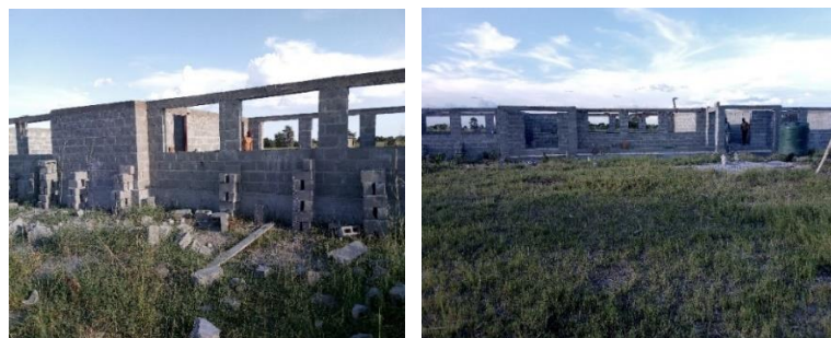
Uncompleted 1x3 CRB at Nalwamba Community School
