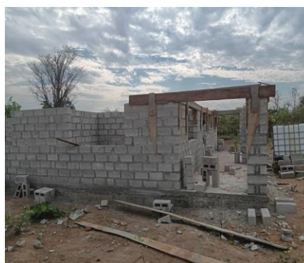
Ring beam being constructed
