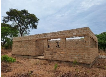
Incomplete Kayisaka Health Post at gable level
