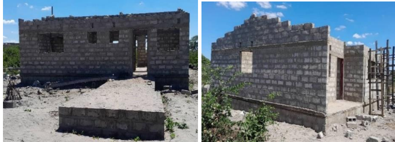
Incomplete staff house
