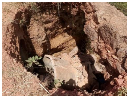
Broken culvert at 8.0 Km
