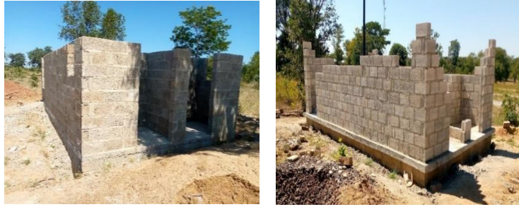
Ablution block 1 and 2 at window level
