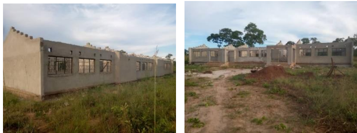
Uncompleted 1 x 3 CRB at Kasheke Community School
