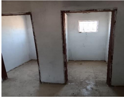
Doors and window not fitted
