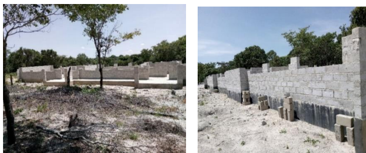
Uncompleted 1x3 Nalinanga Community school
