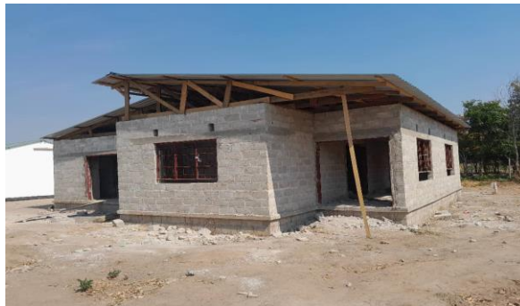
Incomplete theatre block
