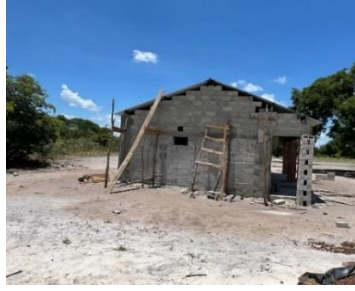
Side view maternity annex
