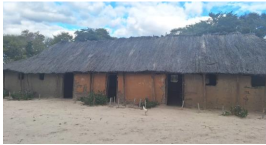
Pole and mud classroom block at Makwaza Community School
