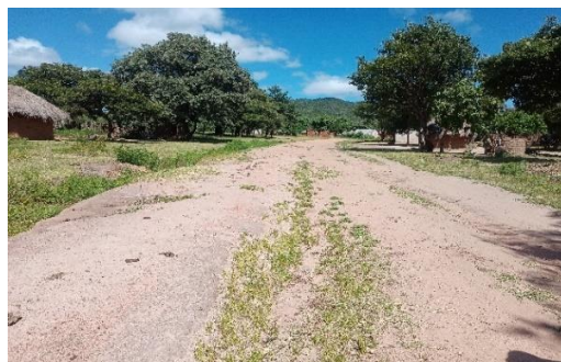
Ungraded and Ungraveled 8 km from start 7.99 km (Ungraded and Ungraveled)
