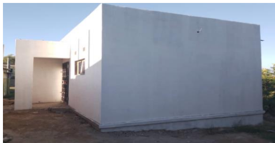
Incomplete Ablution Block at Kariba Secondary School
