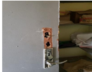
Broken mortice lock
