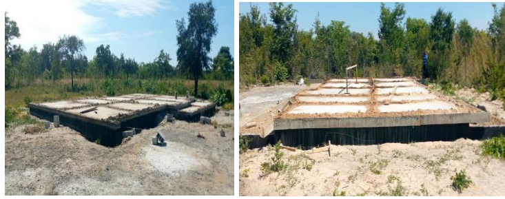
House No. 3 and No. 4 all at slab level
