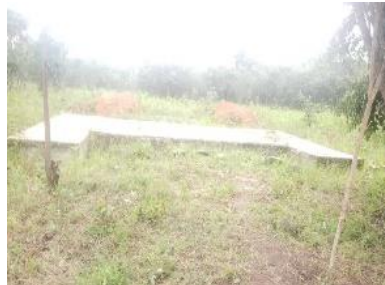
Toilets at slab level
