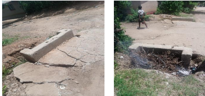
Cracked slab
