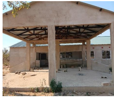
Incomplete floors and ceiling board
