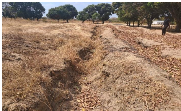
Buried Footing Trenches for a 1x3 Classroom Block
