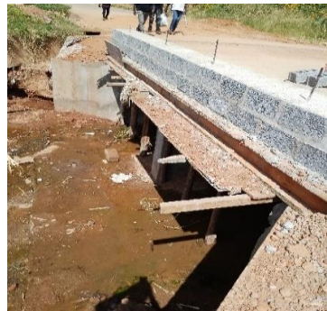
Dambo road Culvert under construction
