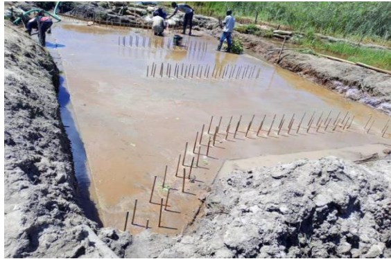
Incomplete Bridge at Chitete stream
