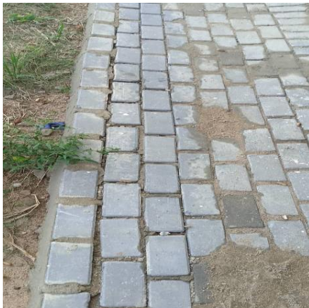
Separating paver bricks
