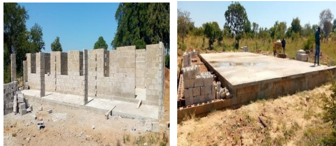
Dormitory at ring beam and dormitory at slab level – Nyawa Secondary School
