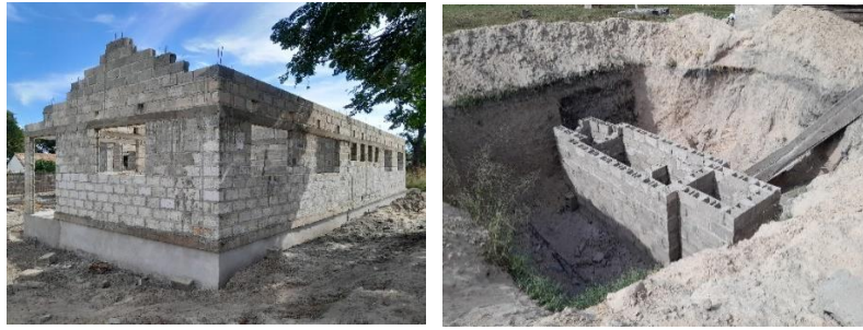
Uncompleted Mothers Shelter at Mangango Hospital
