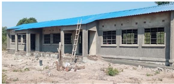
Uncompleted 1x3 CRB at Kafwasonyi Community School
