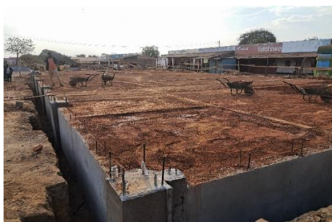
Transit Bus Station at Backfilling Stage
