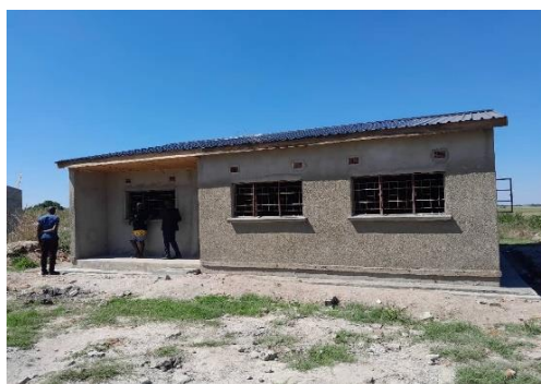
Incomplete staff house
