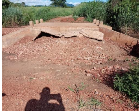
Washed away stone pitching areas of the Constructed Gondar Bridge
