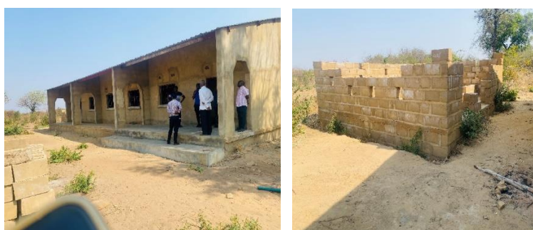
Incomplete Dormitory and Ablution
