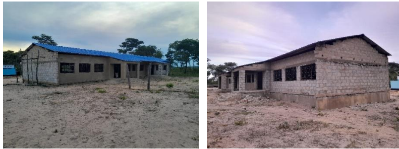
Uncompleted 1x3 CRB at Kachakala Community School
