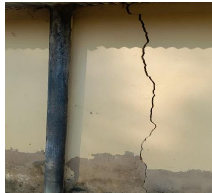
Dilapidated pit latrine being used
