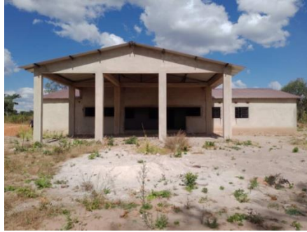
Incomplete Rural Health Post
