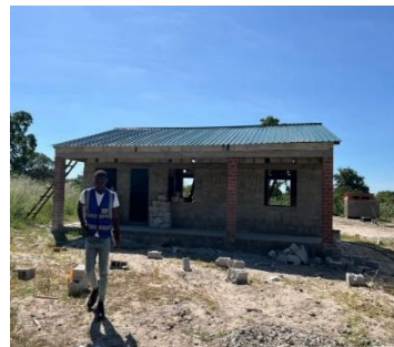
Front view luandui maternity Annex
