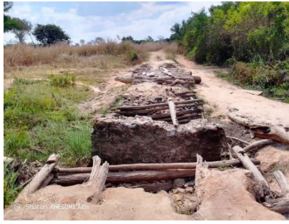
Construction site for Kabisha Bridge
