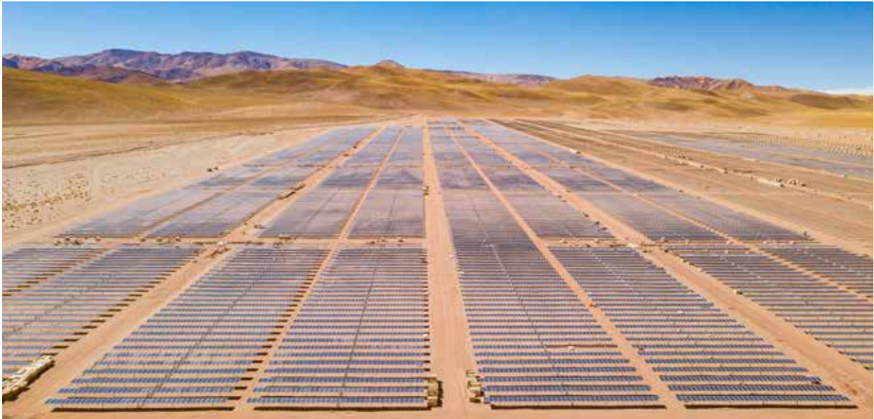
Photo: Aerial view of Cauchari solar project, one of the largest photovoltaic (PV) solar power projects in South America, located in Jujuy, Argentina. Credit: Estebran, Shutterstock.
