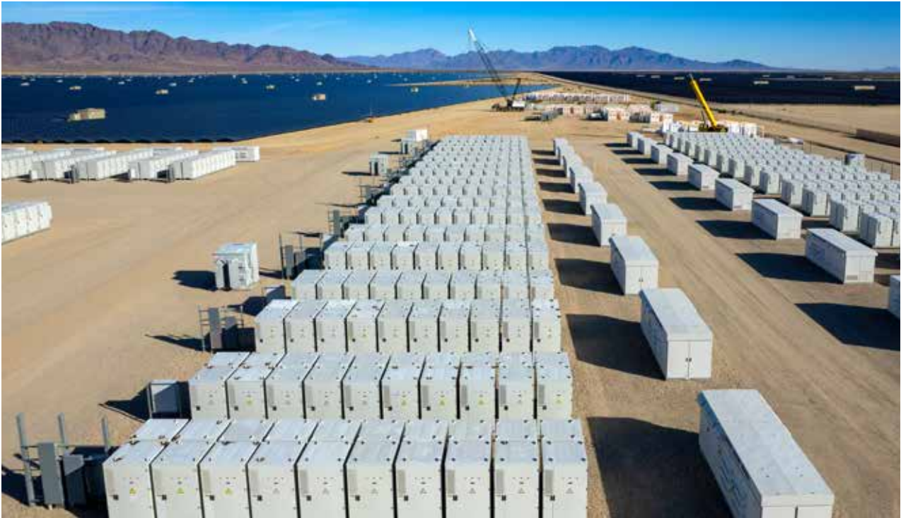
Photo: Aerial view of industrial battery units storing electricity in California, USA. Credit: The Desert Photo, iStock.
